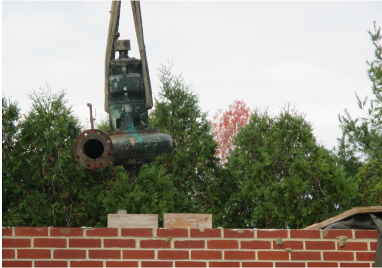
Pump Replacement at a Sanitary Sewer Pump Station
