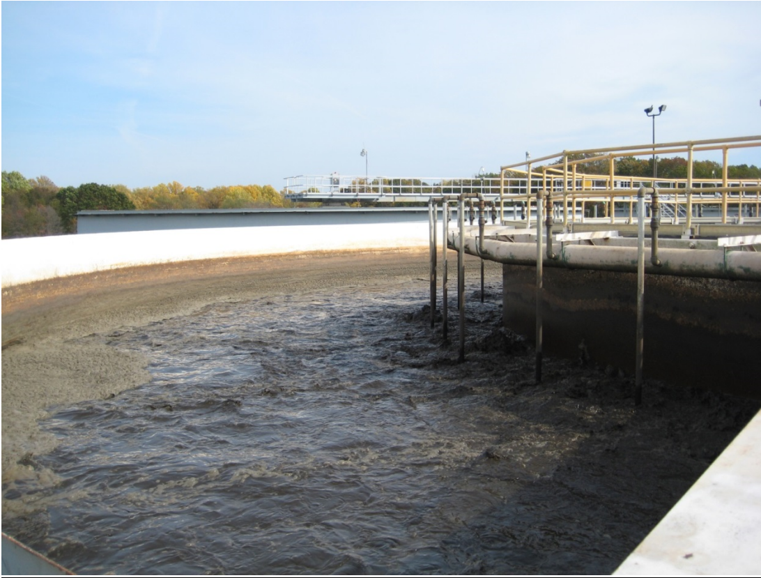
Biosolids Thickener Tank
