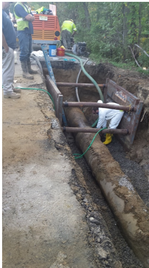
Repairs of Primary Force Main on Elbo Lane
